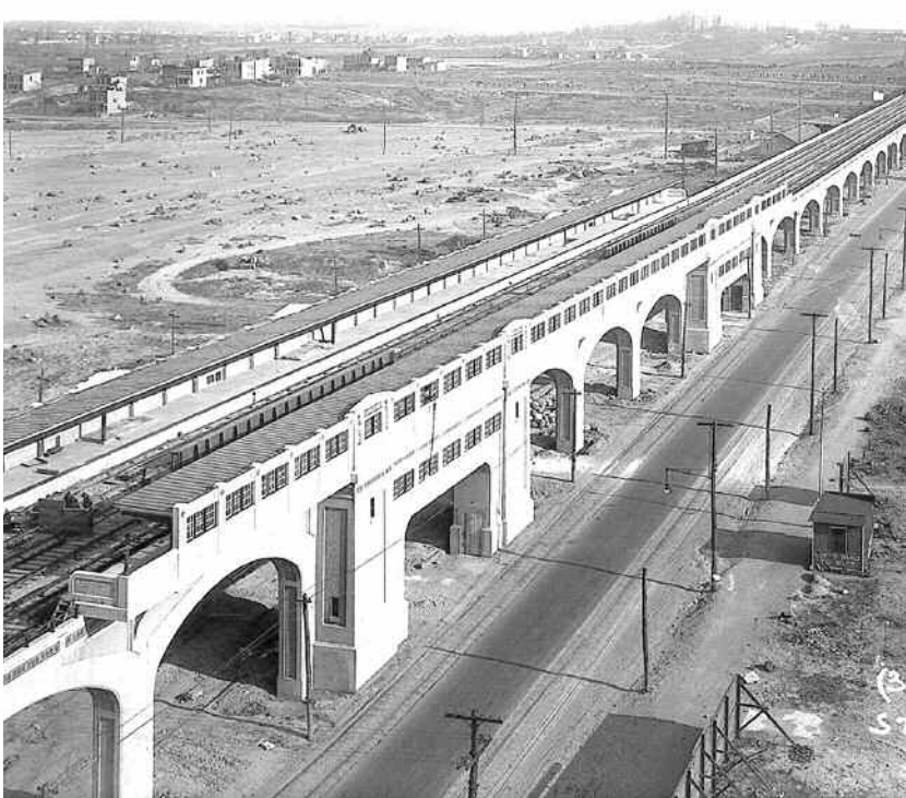
The extension of the Flushing Line along Queens Boulevard, shown at Rawson Street in 1917, completely changed the rural landscape of Queens, spurring intense residential, commercial, and industrial development.
